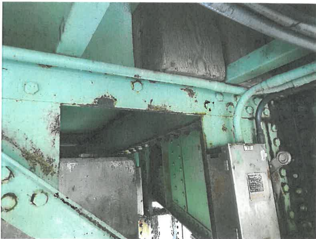
FIXED SPAN 3 - REPAIR SECTION AT FB6 TRUSS (LOOKING WEST)
